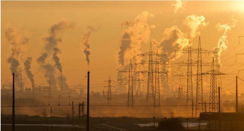
Coal Power Plant. [13]
